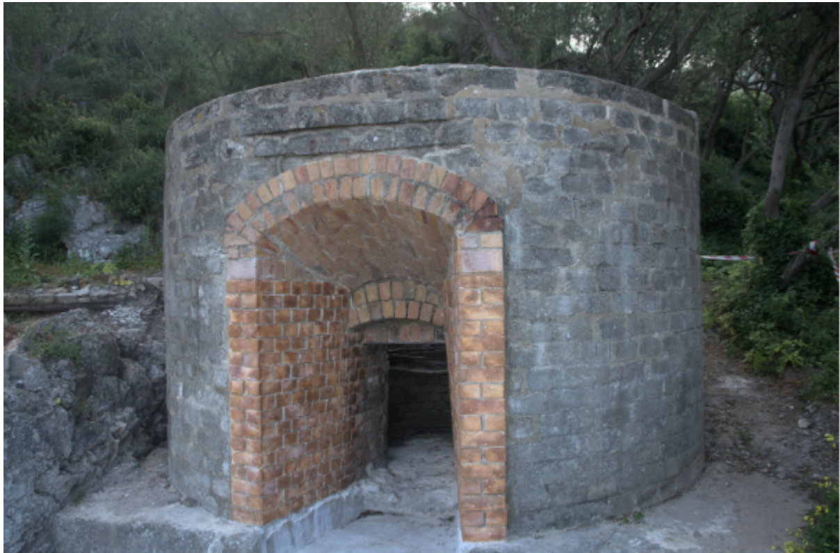
The restored later 19 th -century lime kiln in Willis's Road. It is one of two such kilns located on either side of Gibraltar's Western and Eastern slopes producing quicklime used in the construction of Gibraltar's underground reservoirs and water catchments carried out during the late 19th Century and early 20th Century.
